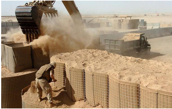
Fig. 4: Installation of Hesco barrier [19]
